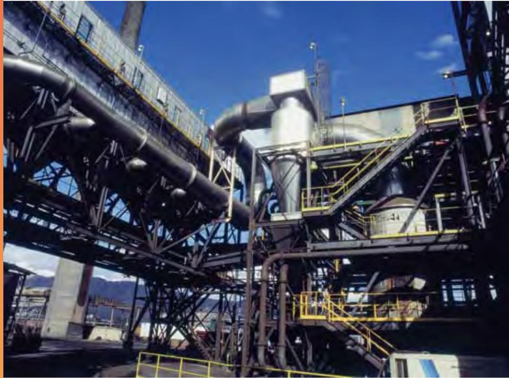
Fluid Bed Dryer Used for Copper Concentrate
